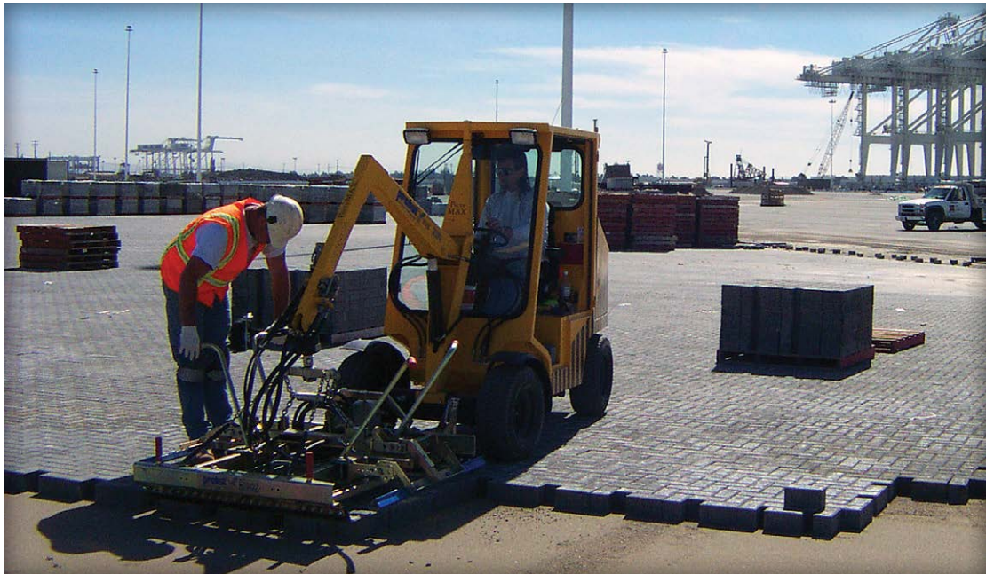
Figure 8. Mechanical installation equipment places concrete pavers rapidly.
