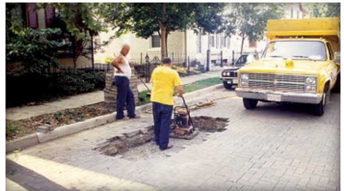
Figure 3. Compaction of the base
