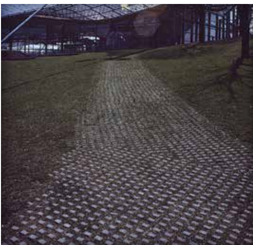
Figure 6. Service access lane
