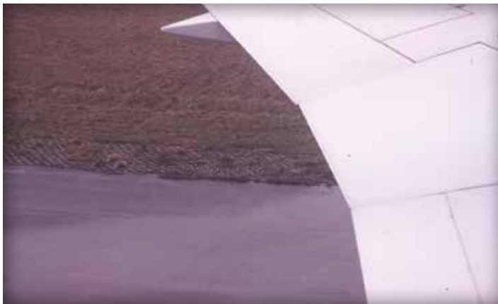
Figure 11. Airfield taxiway shoulder
