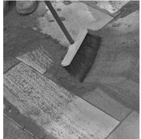
▲ Sweeping sand in the joints
