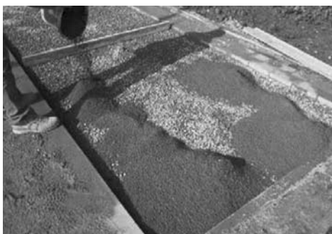
▲ Preparing the setting bed
