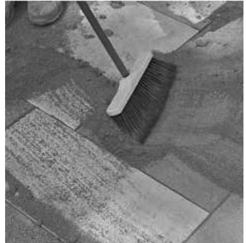
▲ Sweeping sand in the joints
