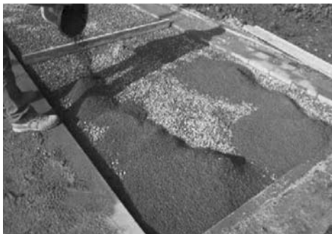
▲ Preparing the setting bed
